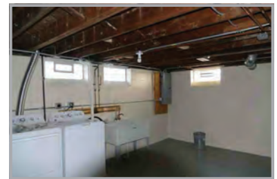
LAUNDRY IN BASEMENT
