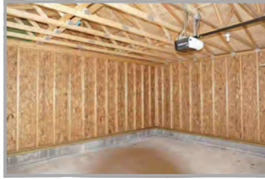
INTERIOR OF GARAGE
