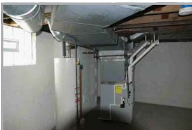
new furnace/new hot water tk
