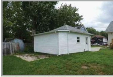
rear of detached garage
